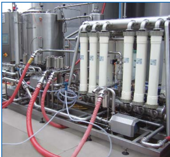
Oenoflow HS-12A System at Chilean winery
